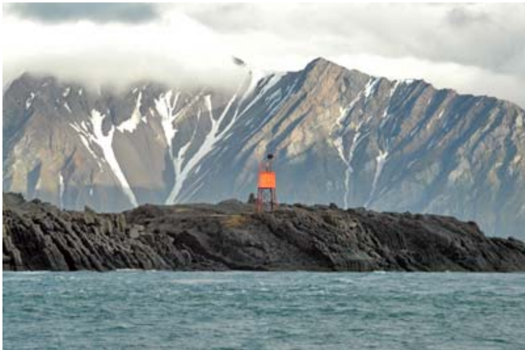
Courtesy of Olav Haugen, Norwegian Mapping Authority Akseloya Light from NW
