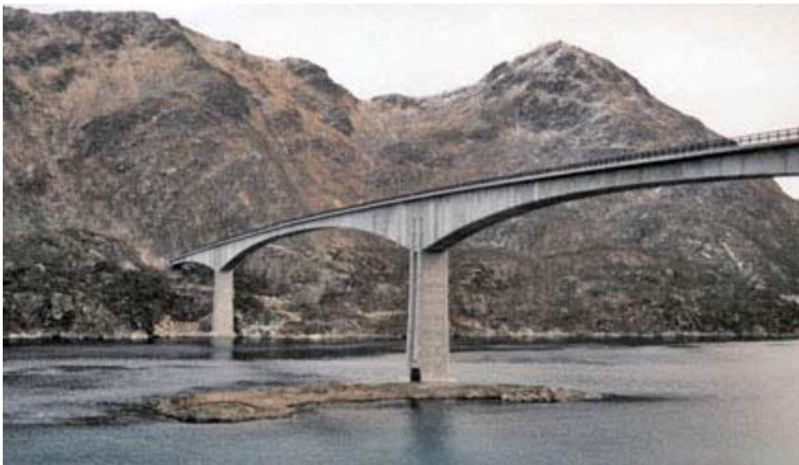
The Raftsundet Bridge from S
