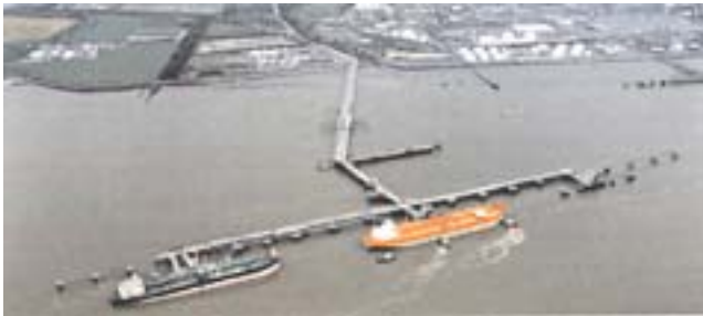
Immingham Oil Terminal
