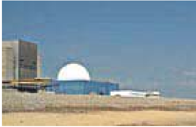
Sizewell Nuclear Power Station
