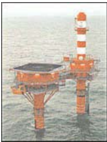
Oostdyck Radar Tower
