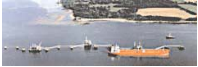
Hound Point Marine Terminal
