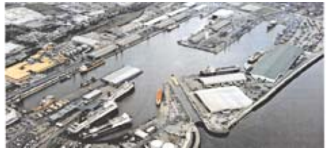
Hull—King George Dock and Queen Elizabeth Dock
