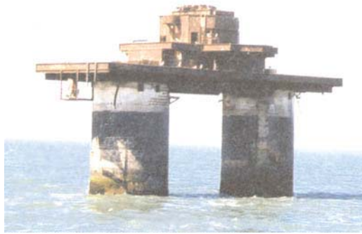
Knock John Tower
