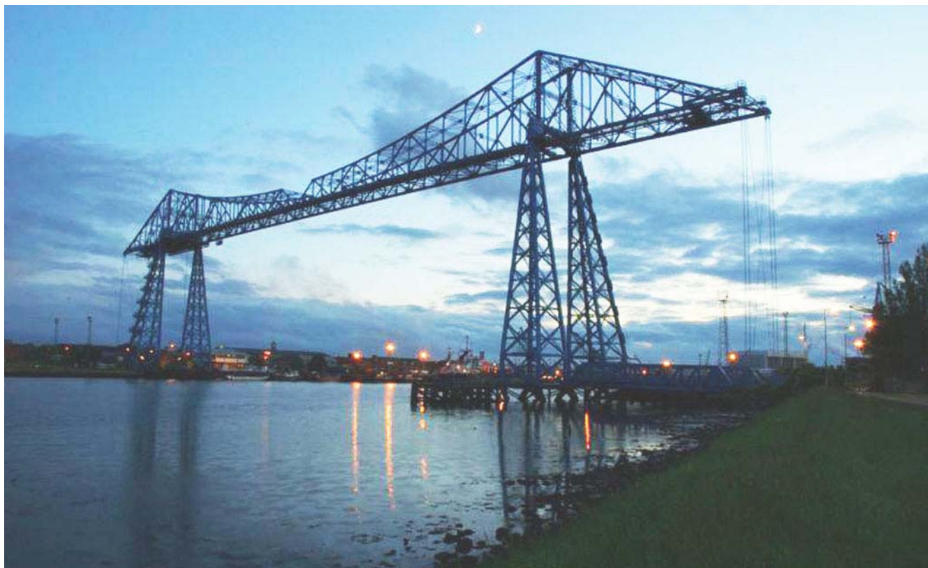
Tees Transporter Bridge
