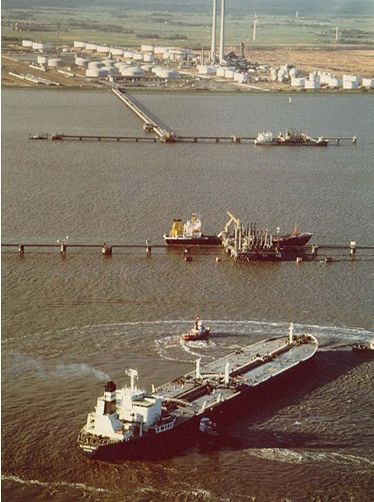
Wilhelms WRG Terminal
