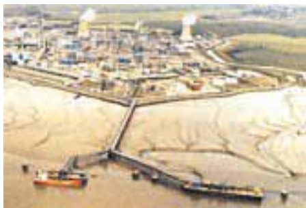
Salt End Oil Terminal
