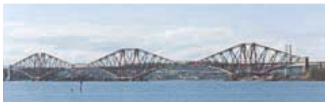
The Forth Bridges from NE
