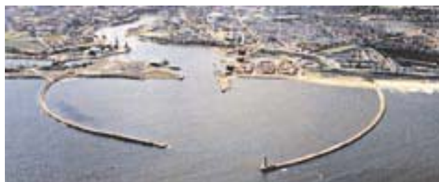
Entrance to the River Wear (Sunderland)
