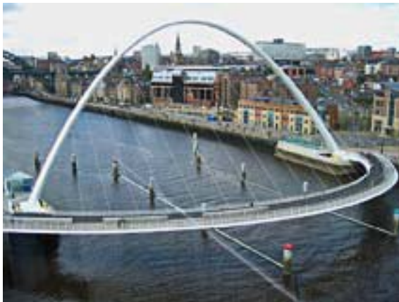
Gateshead Millennium Bridge (closed)
