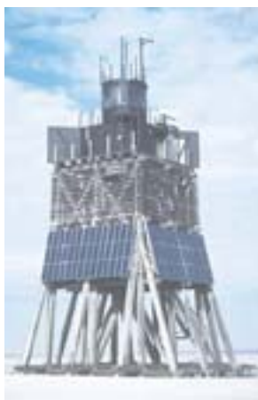
Suderoogsand Light (Refuge Beacon)
