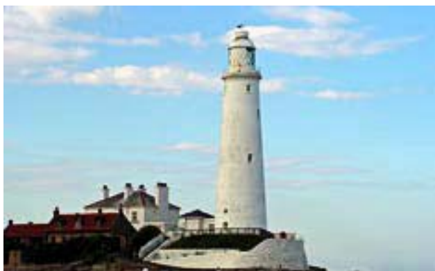
St. Mary's Island Disused Lighthouse
