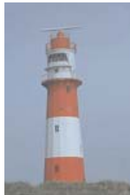
Borkum Little Disused Light Tower
