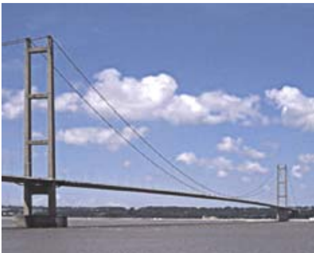
The Humber Bridge
