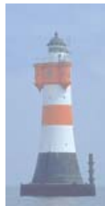
Roter Sand Tower
