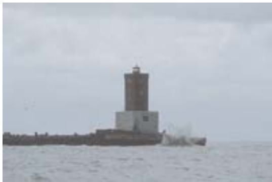
Minsener Oog Disused Light Tower (Buhne A)
