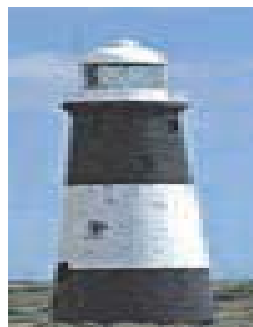
Spurn Head Lighthouse (disused)
