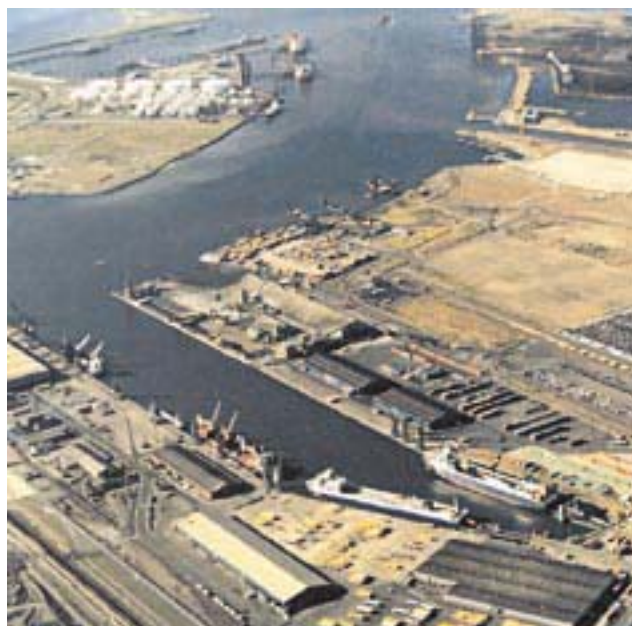
Tees Dock and Norseia Oil Terminal
