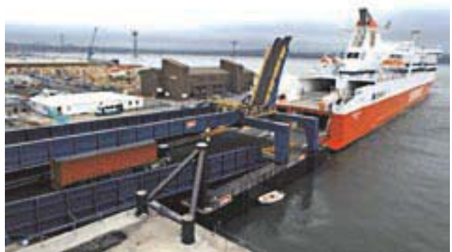
Rosyth Ferry Terminal
