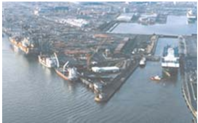
Bremerhaven—Nordschleuse (North Lock)
