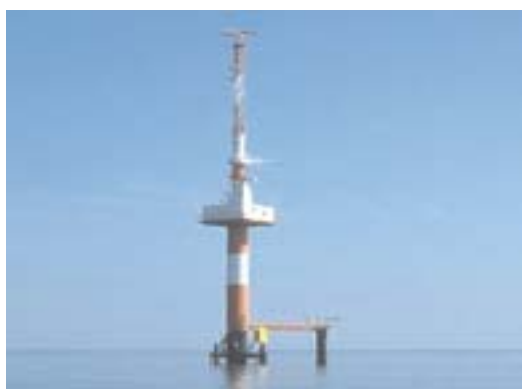
Hooksielplate Radar Tower
