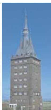
Wangerooe West Tower
