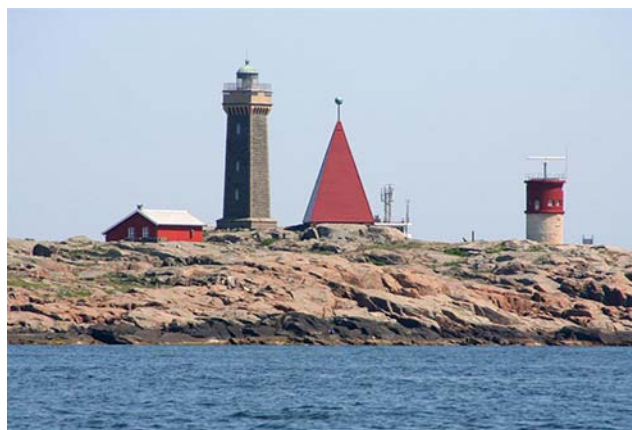
Vinga Light, day beacon, and radar tower
