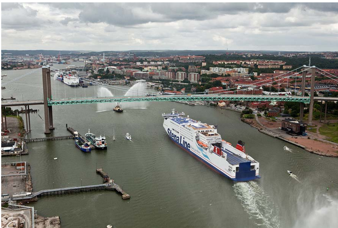
The Alvsborg Bridge (Goteborg) with the Dalanas Pier and the Ryahammen Pier on the Left
