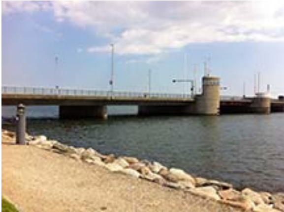
The Hadsund Bridge
